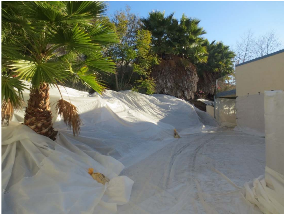
Photo 2: Pre- excavation: Plastic laid down along soil transport route, north of Building G.
