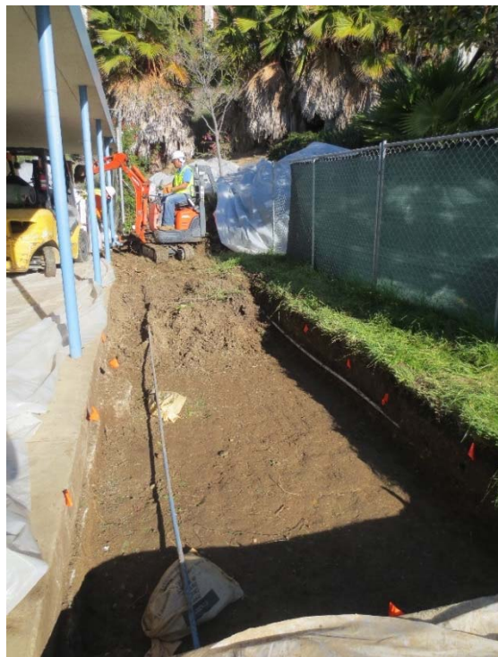
Photo 14: Second day of excavation: Completing northern half of excavation while southern half is flagged for incremental sampling.
