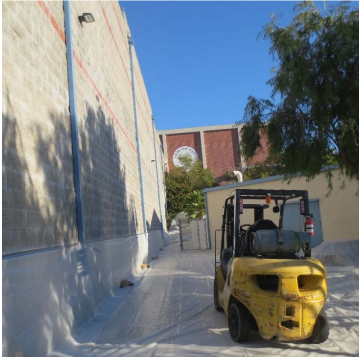
Photo 1: Pre-excavation: Plastic laid down along soil transport route, east of Gymnasium.
