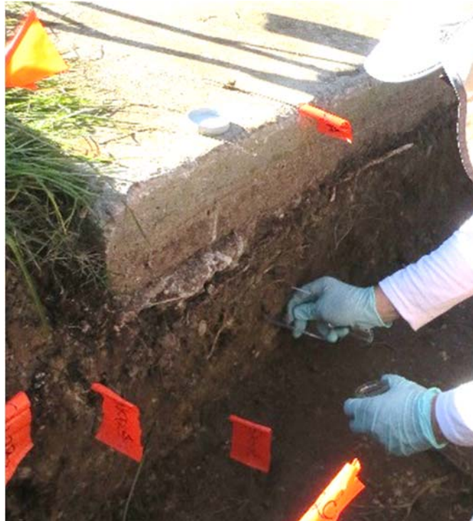
Photo 17: Collecting southern sidewall post-excavation incremental soil sample.
