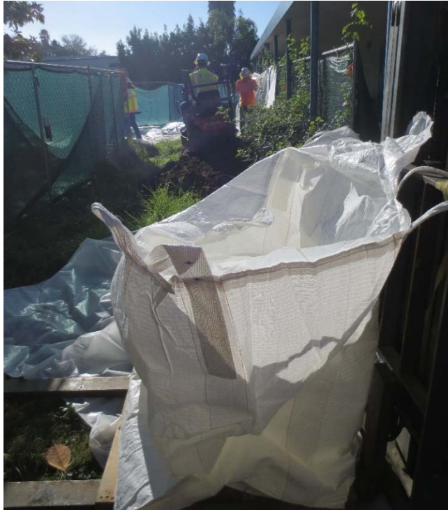
Photo 9: First day of excavation: Empty Super Sack® loaded on forklift, looking south.
