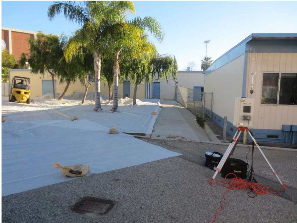
Photo 3: Pre-excavation: Setting up air monitoring station (ENVIRON), looking east toward Building G.
