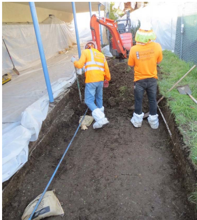
Photo 12: First day of excavation: Southern end of excavation down to total depth of 1.5 feet; blue irrigation line supported by sandbags.
