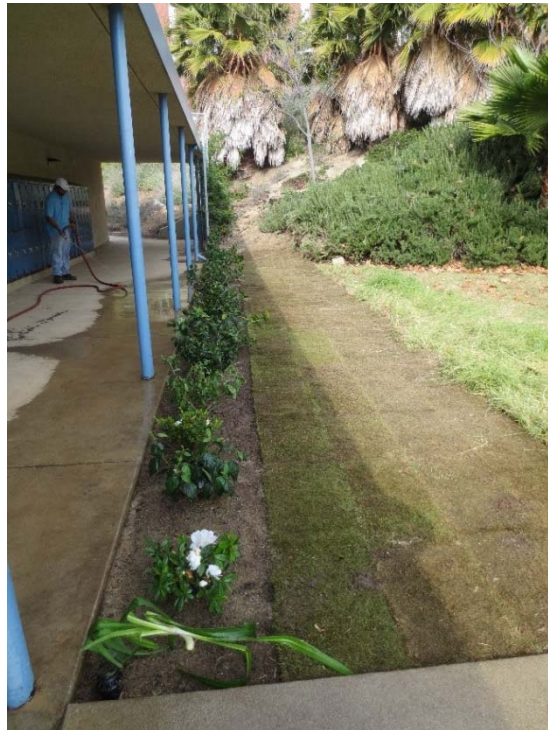
Photo 20: Post Excavation: Looking north - Excavation area restored to previous state with sod and plants.
