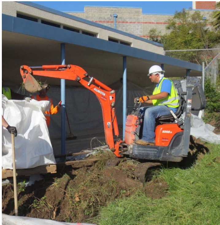
Photo 10: First day of excavation: Loading excavated soil into Super Sack®; lockers covered in plastic in background.
