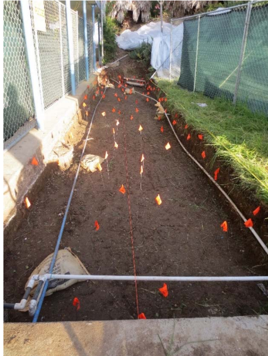
Photo 15: Completed excavation with flagged post-excavation sampling locations, temporary fencing, and plastic; looking north.
