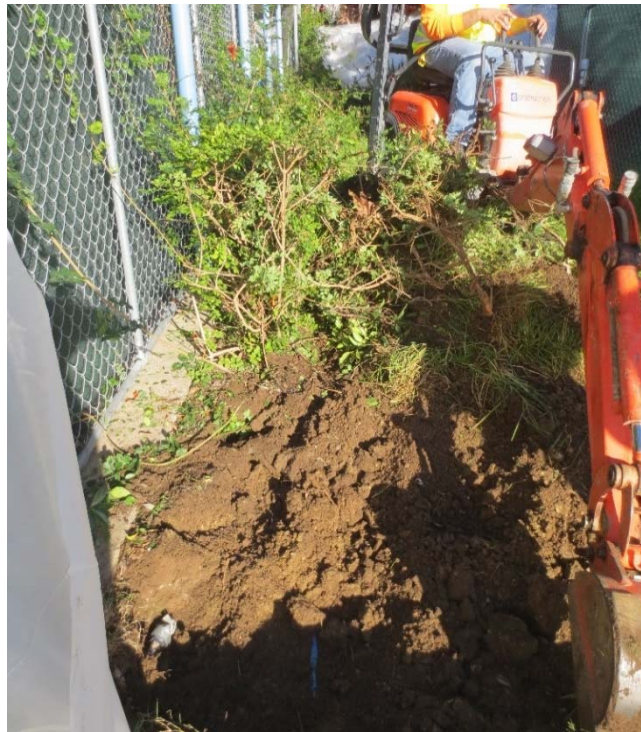
Photo 8: First day of excavation: Removing shrubbery adjacent to walkway; irrigation lines (blue, gray) exposed.
