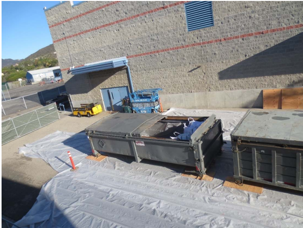
Photo 13: Second day of excavation: Roll-off bins staged on plastic by Gymnasium, looking northwest.
