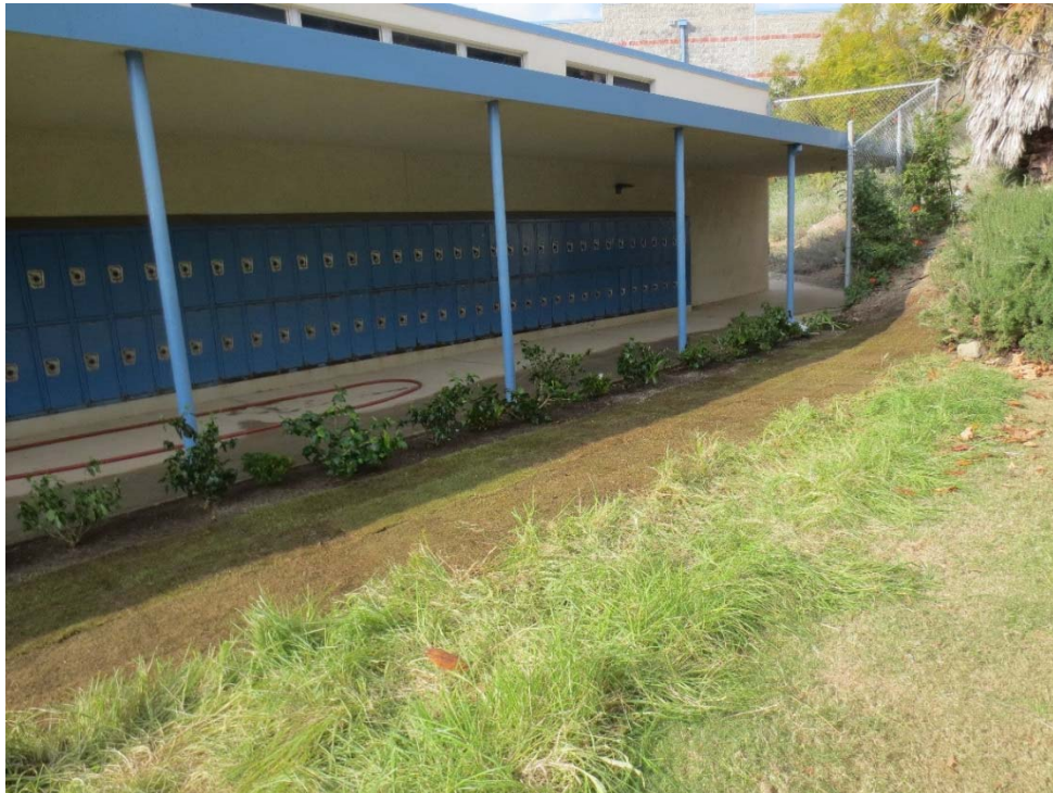
Photo 21: Post excavation: Looking northwest - Excavation area backfilled and restored.
