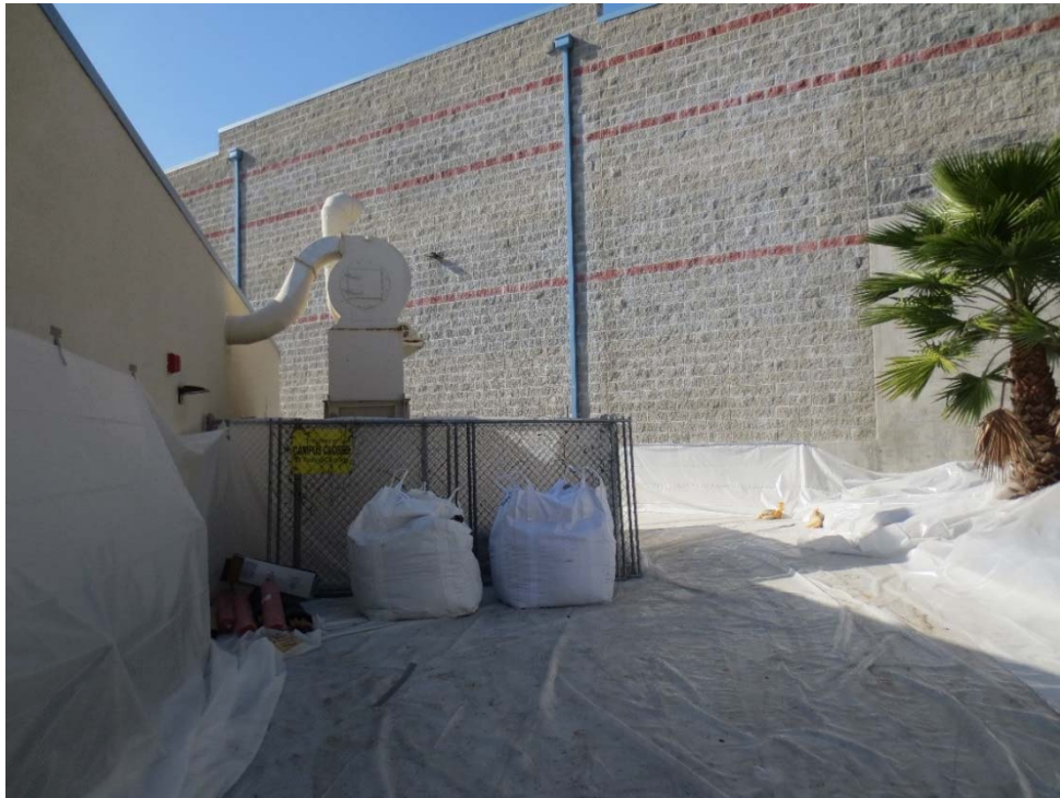
Photo 11: First day of excavation: Temporary Super Sack® staging location north of Building G; plastic sheeting on ground, walls, and hill.
