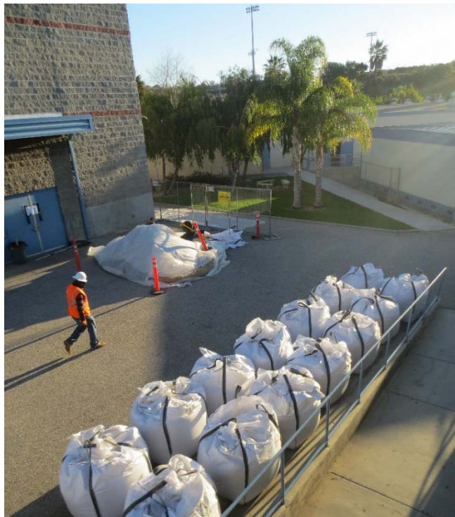
Photo 18: Looking east at Building G: Staging area for Super Sacks of clean imported soil for backfill (to the right) and stockpile of imported topsoil covered in plastic (to the left). Note that the fill soils were approved by DTSC.
