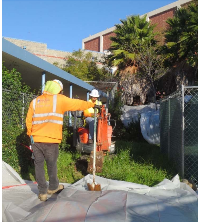
Photo 7: First day of excavation: Removing grass and surficial soil with mini-excavator, looking north.
