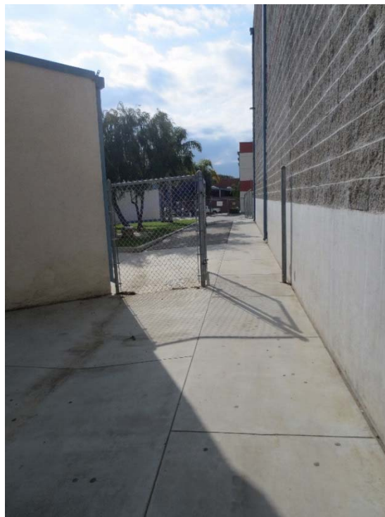
Photo 22: Post excavation: Looking southwest: Soil transport route adjacent to Gymnasium after excavation activities.
